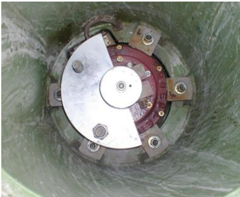
Image 1: Direct drive; driveshaft through motor.
