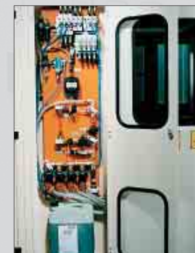
Pneumatic controls, process water and compound dosing system
