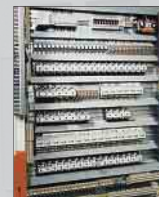
State of the art controls
