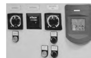
Electrical controls and compound dosing
