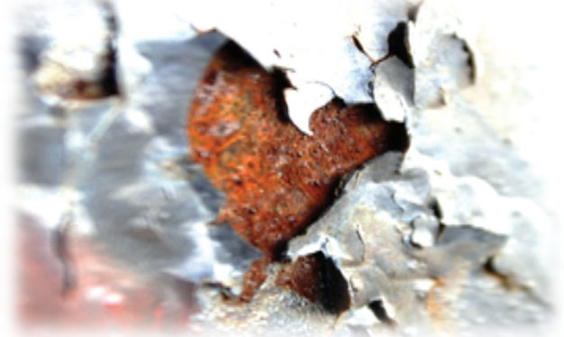
Rust under Paint
