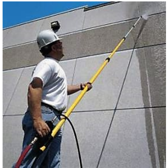
Exterior Building Surfaces
