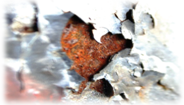
Rust under Paint
