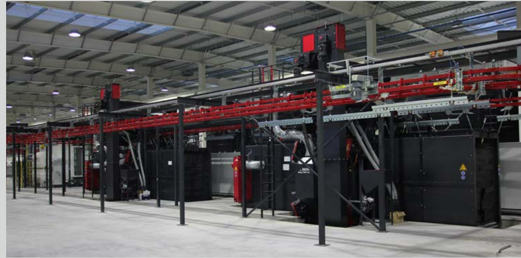
The work pieces are passing through two identical, sequentially arranged hanger machines for blast-cleaning and subsequent shot peening.
