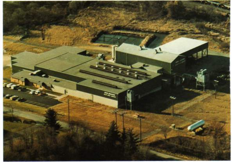
AMASTEEL Plant, Butler, Pennsylvania
