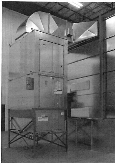
Vertical indoor side discharge
